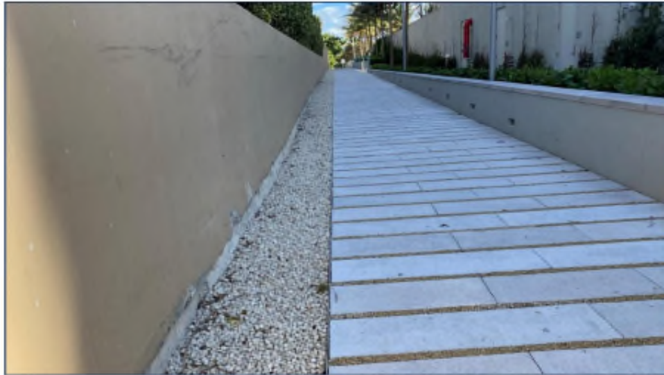
Figure 1: South Perimeter Wall (left) and beach access path (right)
